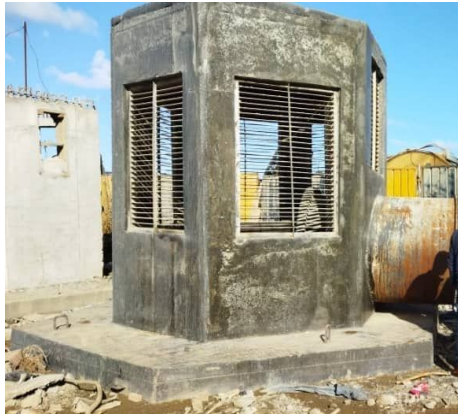
a) Water intake tower
