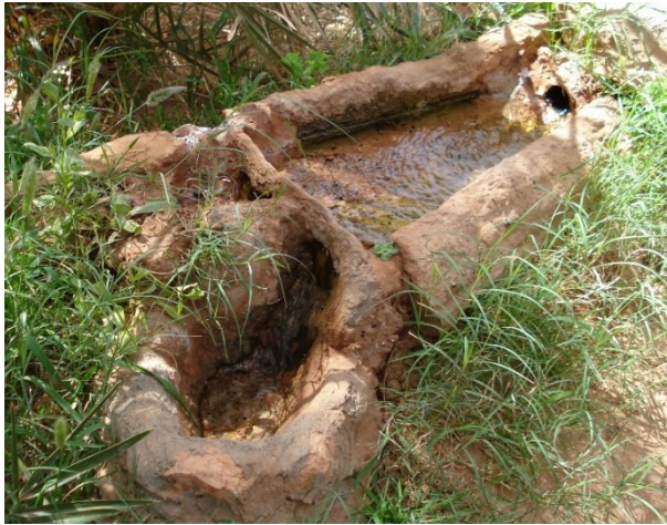
Figure 10: Kasria of a foggara in Timimoun. For more than 20 centuries, approximately 1000 foggaras have been exploiting the waters of the Continental Intercalaire aquifer (Photo. Remini, 2008).
