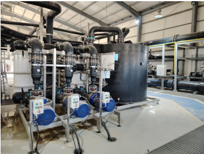
Figure 14: El Oued demineralization station for brackish waters from the Continental Intercalaire aquifer (Photo. Remini, 2023)
