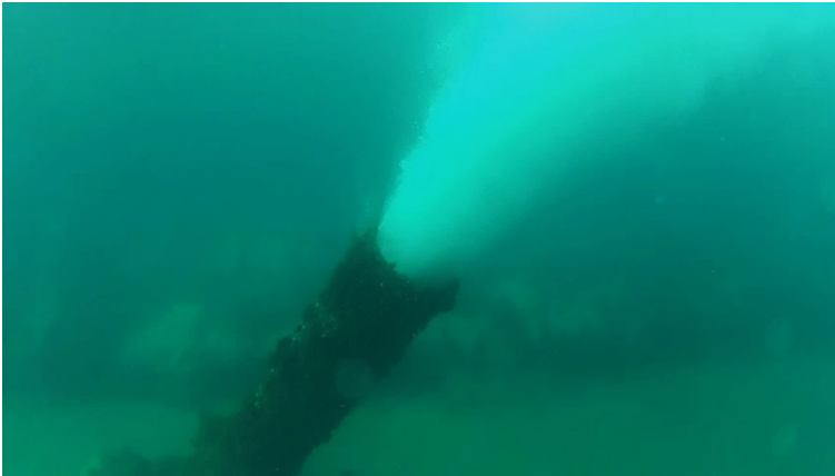
Figure 19: Direct discharge of brine into the seabed from a desalination plant in Algeria (Fouka Station) (Remini and Amitouche, 2023a).
