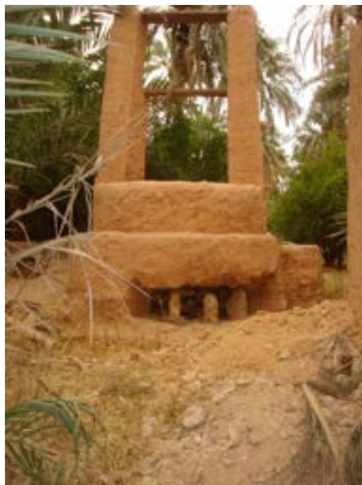
Figure 40: Diagram of a traditional well designed to slowly recharge groundwater (Photo Remini, 2014)
