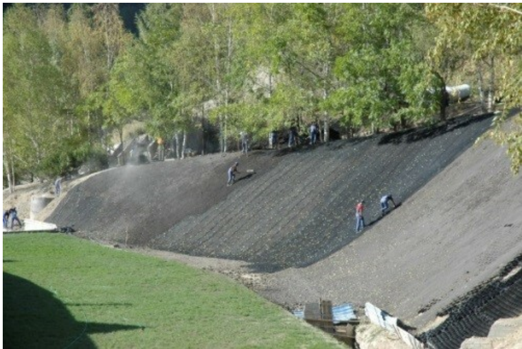
(b) Photo 2: Slope reinforcement using geomat, (a) for the reinforcement of road drainage channels; (b) with a biological type of reinforcement
